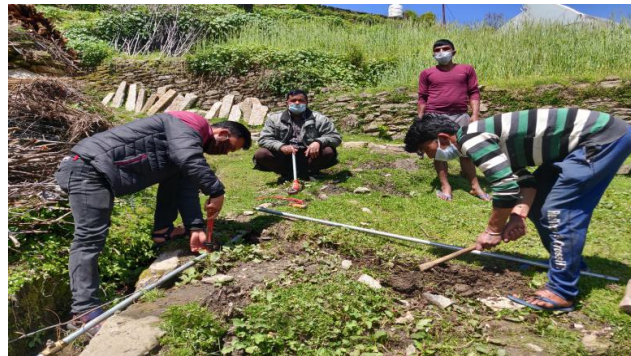
Pipeline fitting work in village Wachham
