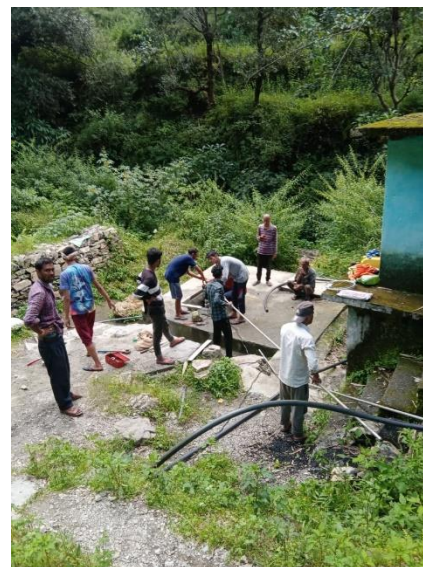
Preparations for solar lift scheme in Pali village, Pauri Garhwal
